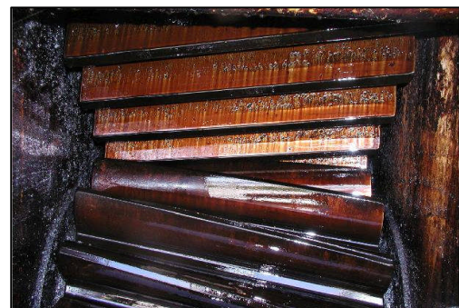
North side of kiln girth & pinion gear set showing lubricant coating after setting idle
